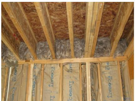
Bonus room floors, cantilevers, and floor insulation have no chance of performing since the insulation is not installed in permanent contact with the subflooring.
