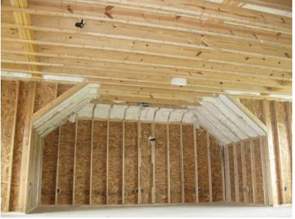
Wind Intrusion – wind blows through the insulation and reduces its R-Value. Hard-decking, "wind tunnels", or foam prevents this.
