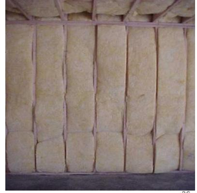
Misalignment – insulation must be touching the air barrier to work correctly. For example, skin is our air barrier. A blanket 12" away will not keep us warm, either.
