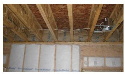
Only spray foam insulation works as both an insulator and air barrier. F/G batts and cellulose allow unconditioned air to flow through it and this leads to energy losses, nail pops, and trim cracks.
