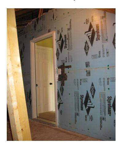
If 990sf of an attic has perfect R30 insulation but the 10sf of attic access is uninsulated and unsealed with an R1 the total R Value is R23.
