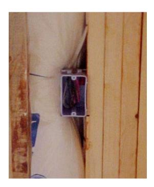
Voids – when insulation is missing entirely. The blower door and infrared camera help identify these areas.
